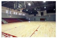
lighting patterns for the gym floor. The ultra-high efficiency driver (ballast) is available in **110V~277V or 310V~520V** autosensing and **50hz/60hz** to meet U.S. and European standards. Mercury is a solid encapsulated amalgam, making Gym-Bright<sup>TM</sup> environmentally friendly and safe. No special handling is required. No hazardous material disposal is necessary. But, with 100,000 lifecycle, most will last up to a century! Available in glass or polycarbonate.
